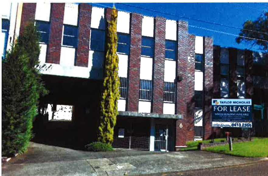
Figure 11. Vacant large format office - industrial property in East Chatswood
